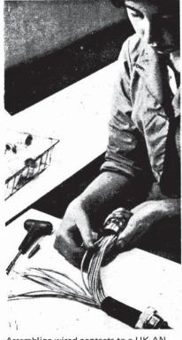
Assembling wired contacts to a UK-AN connector.
